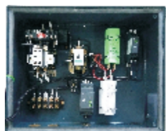
Interior View of MR-G2W
