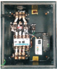
Interior View of MU-G10W DOL
