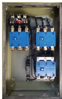
Interior View of ML FASD
