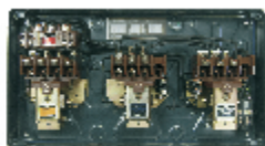
Interior View of MK2 FASD
